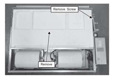
2 Unscrew 5 screws on the Evaporator and remove 2 sensor from holder and remove Evaporator from the unit.
